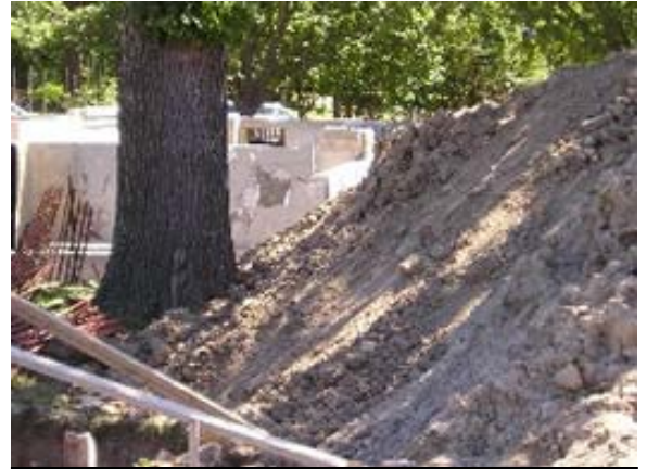
Soil compaction results from storing materials under a tree
