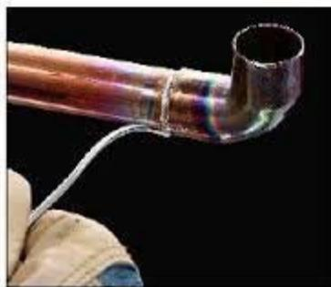
Solder made of 50% Lead & 50% Tin was used in joining copper pipes until banned by the 1986 Federal Safe Drinking Water Act. This is not a major contributor to drinking water lead for a couple of reasons.
